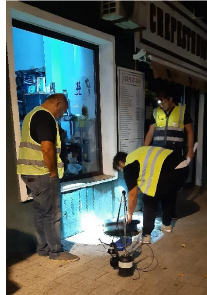
Development of active leakage detection as a daily activity to find invisible bursts
