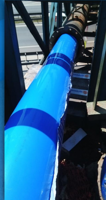
AFTER PULLING MATERIAL
