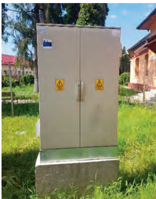
Fig. 7. Foraj Valea Mare / Valea Mare Drilling
