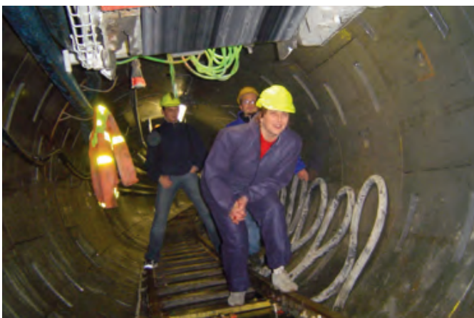
Fig. 3. Colectorul Iașilor realizat prin scut / Iasi collector made by shield
